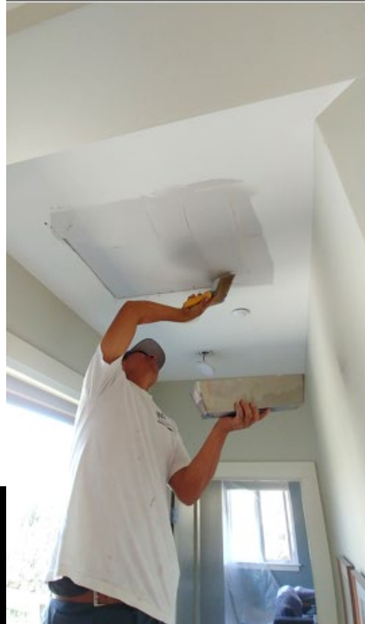
Removal and drywall patching of legacy vents.
